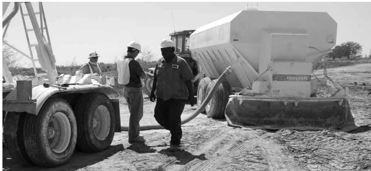
Figure 14. Material Loading onto Spreader
