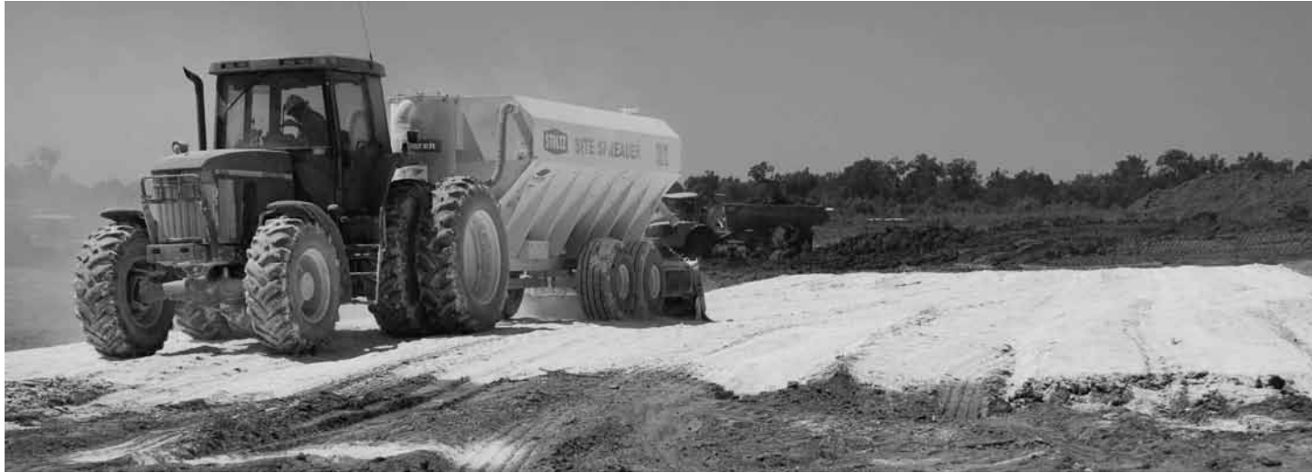
Figure 15. Lime Spreader Depositing Material
